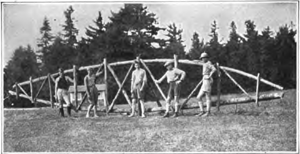
ONE SIDE OF THE SECOND SPAN (30 FOOT) COMPLETE
